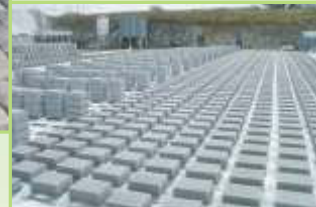
Rigid and Hollow Cement Block Manufacturing Work
